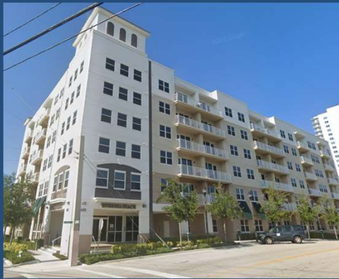
Evernia Place 85 units =< 80% AMI
